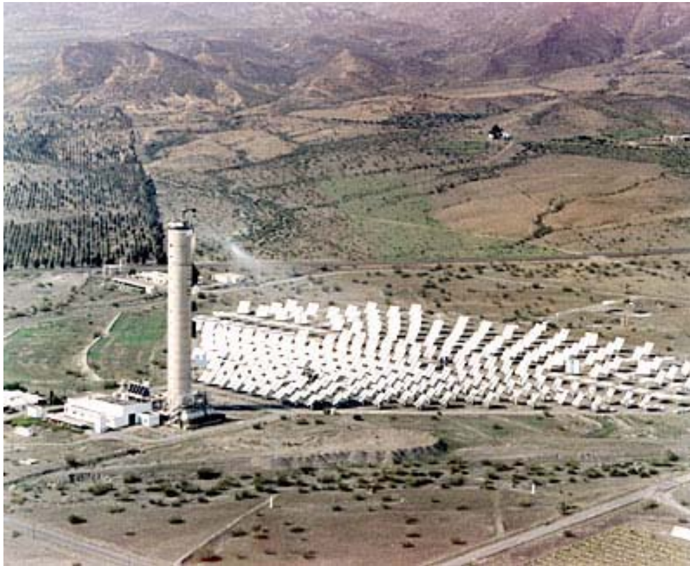
Figure 5. Solar Tower plant in Almeria, Spain.
