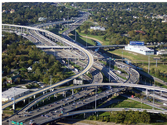
Interstate 10 and Interstate 45 near downtown Houston, Texas in the United States.
