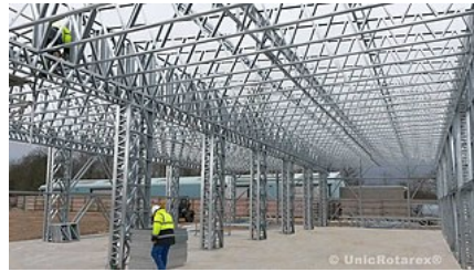
Three dimensional truss construction made by UnicRotarex® ( https://www.unicrotarex.com/metal-truss/ )
