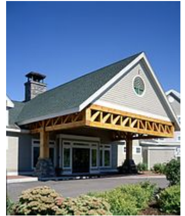
A large timber Howe truss in a commercial building
