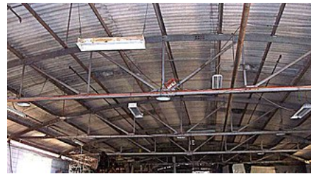
Pre-fabricated steel bow string roof trusses built in 1942 for war department properties in Northern Australia
