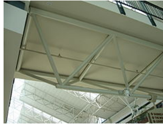
A space truss carrying a floor in The Woodlands Mall
