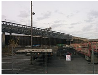
Modern temporary bridge made of Bailey bridge truss panels in Montreal Québec
