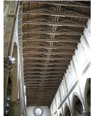
The roof trusses of the Basilica di Santa Croce in Florence
