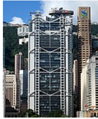
The HSBC Main Building, Hong Kong has an externally visible truss structure
