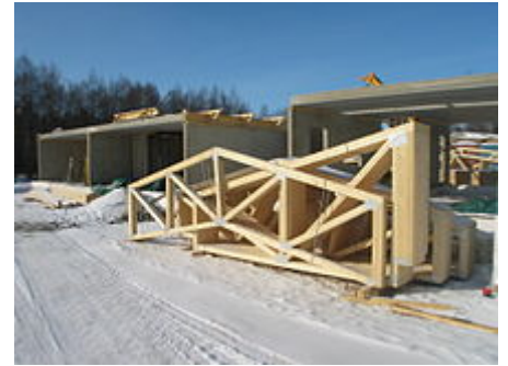
Planar roof trusses
