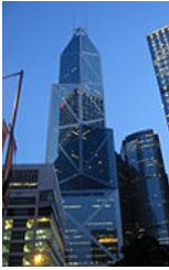
The Hong Kong Bank of China Tower has an externally visible truss structure
