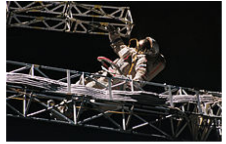
Cosmonaut Alexander Serebrov sets up an integrated truss structure "Rapana" at Mir space station, September 16, 1993
