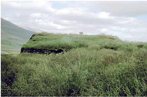
Grass-covered house in Iceland
